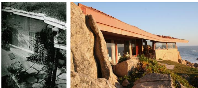
The roof finishing with wooden fascia boards in Villa Mairea and in Boa Nova Tea House. L'Architecture d'aujourd'hui n. 29, 1950, p.23 and photography by Ana Isabel Costa e Silva 2012.
